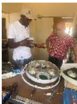
some old and broken theatre lights to use LED bulbs.
