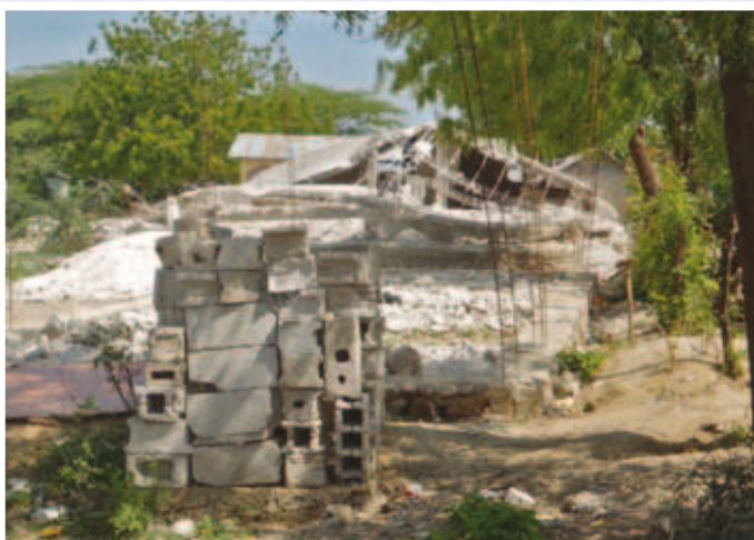
La Tremblay church after the earthquake
