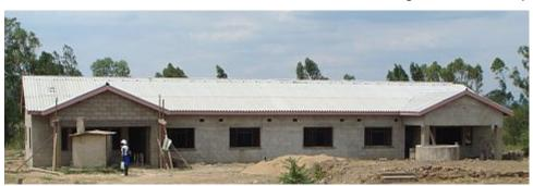
supply. Bath tubs are waiting to be fitted and other plumbing is yet to be finished. Light fittings and switches, and so on, are not yet in place and the windows are not yet glazed, and then there will be painting to be done, but they are confident that all of that will be completed in the next three weeks. Then we will hold an opening ceremony. All in all it is a much happier situation than last year when we wondered if we would manage to finish the building at all. Now we
