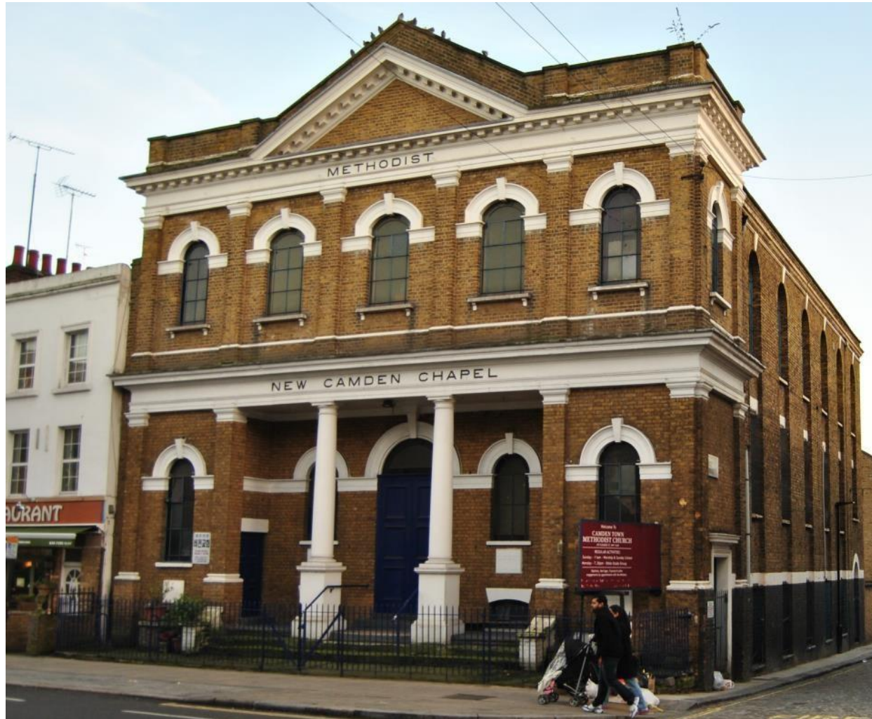
Exterior: Front of the building
