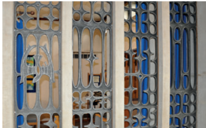
Top: The St. Peter Window, featuring etched episodes of Peter's life with Christ - as fisherman, disciple and apostle. Bottom: Cast aluminium tracery screen which forms the link between the Church and the Lady Chapel
