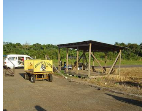
Utila Airport Terminal in good weather.
