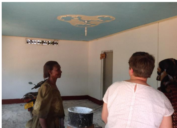
A new manse being renovated at Buyende, Uganda
