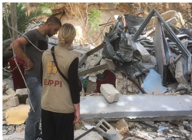
EAs attending a home demolition. Photo credit: EAPPI/EA Michael
