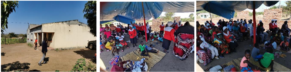
Chimoio Manse. (Built with MCB funds). Chimoio worship in unfinished Church.
