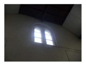
Visits to other churches highlighted a potential solution, which involves secondary glazing units fitted into the window reveal (as illustrated in the image below, taken at Claremount Church). This approach could be applied at Little Neston.
