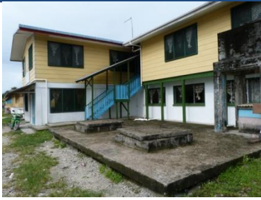
Underground water-storage at the EKT Church Head Office
