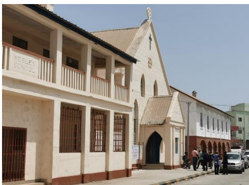
Connexional Office, Banjul, Gambia.
