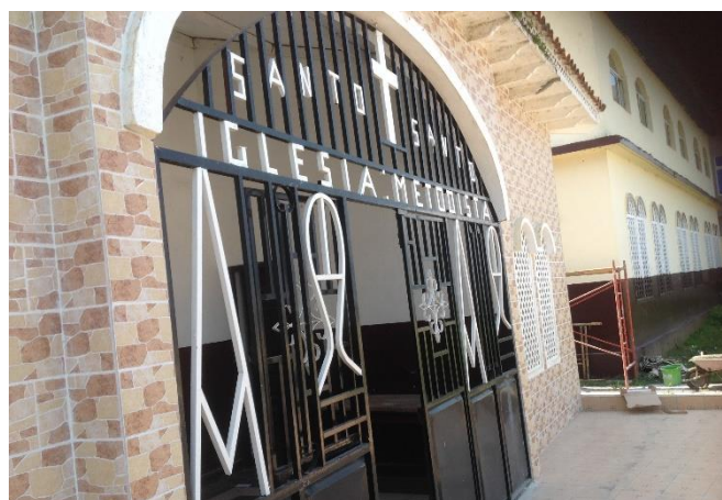
Newly refurbished church entrance
