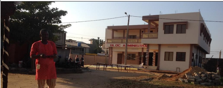
The new GSH administration block built by CeVaa, France
