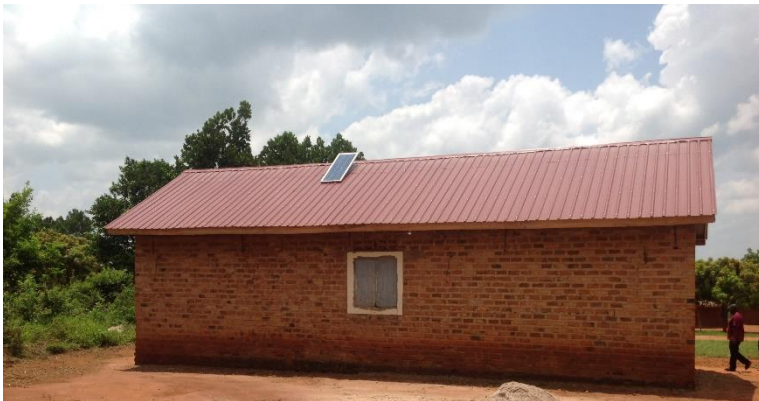
Solar panel for light supply at Buyende Methodist Church
