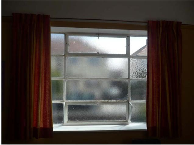
If the condition of the units deteriorates to the point at which significant air infiltration is occurring then the case for replacement becomes more pressing and the payback in terms of energy efficiency will shorten.
